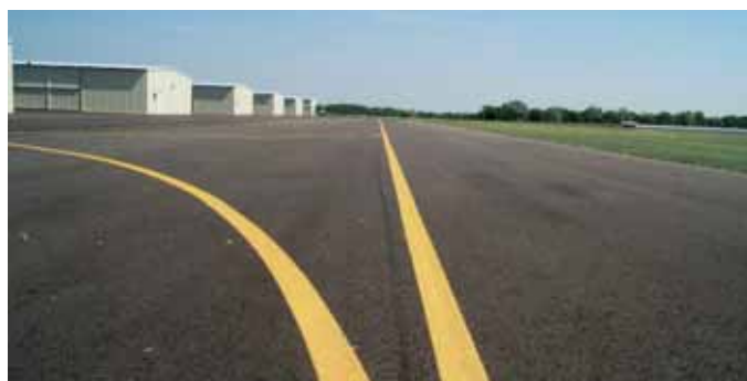
Taxiway markings are yellow. The centerline is a single yellow line, and the taxiway edge is marked by a double yellow line. Dashed edge markings allow the aircraft to cross to the adjoining apron.
