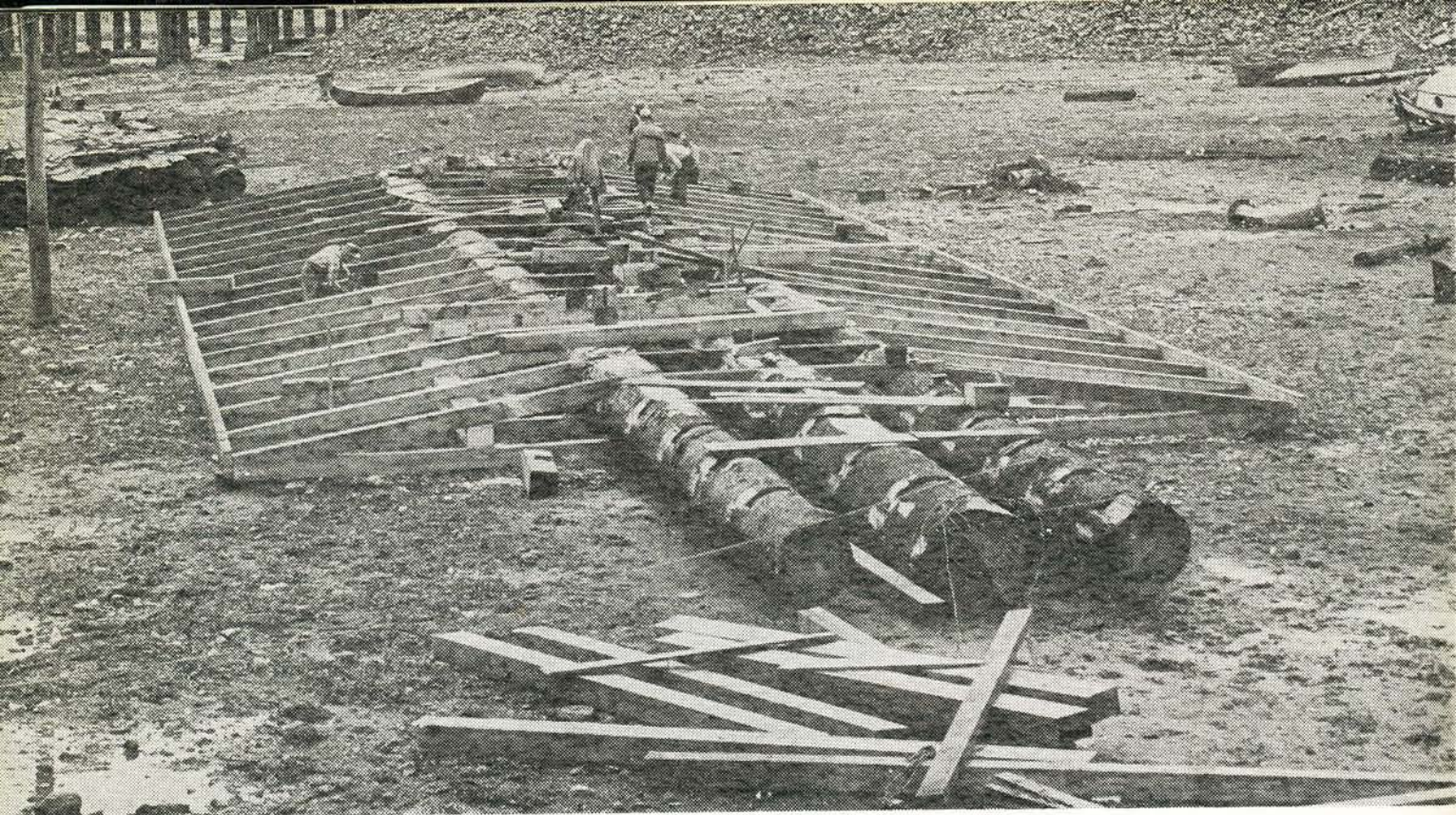
Start of construction on a new seaplane float at Juneau, using local spruce float logs and timbers. The primary structure is built on the beach between high tides which reach a height of twenty-six feet.
